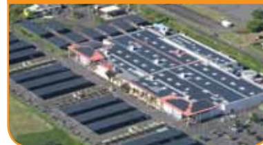
18 MW power plant in La Reunion, France
