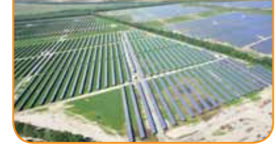
78 MW power plant in Senftenberg, Germany
