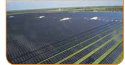
43 MW power plant in Puglia, Italy
