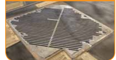
3 MW power plant in Villanueva del Aceral, Spain
