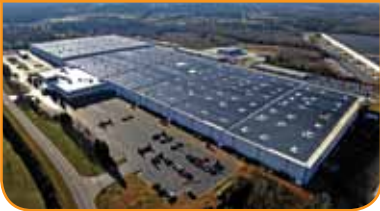
5.2 MW power plant in North Carolina, USA
