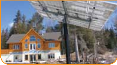
6 kW residential installation in Ontario, Canada
